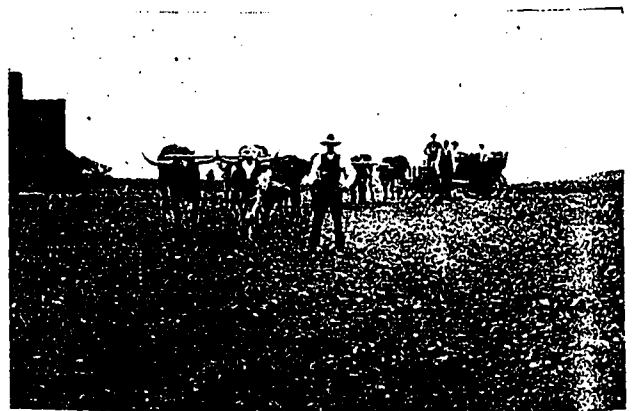
Being Pulled Through Deep Sand with Oxen.
