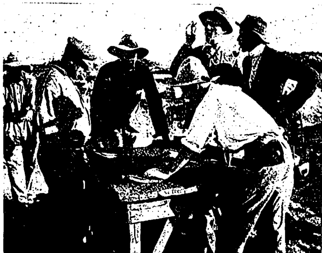
A Diamond Sorting Table at the River Diggings.
