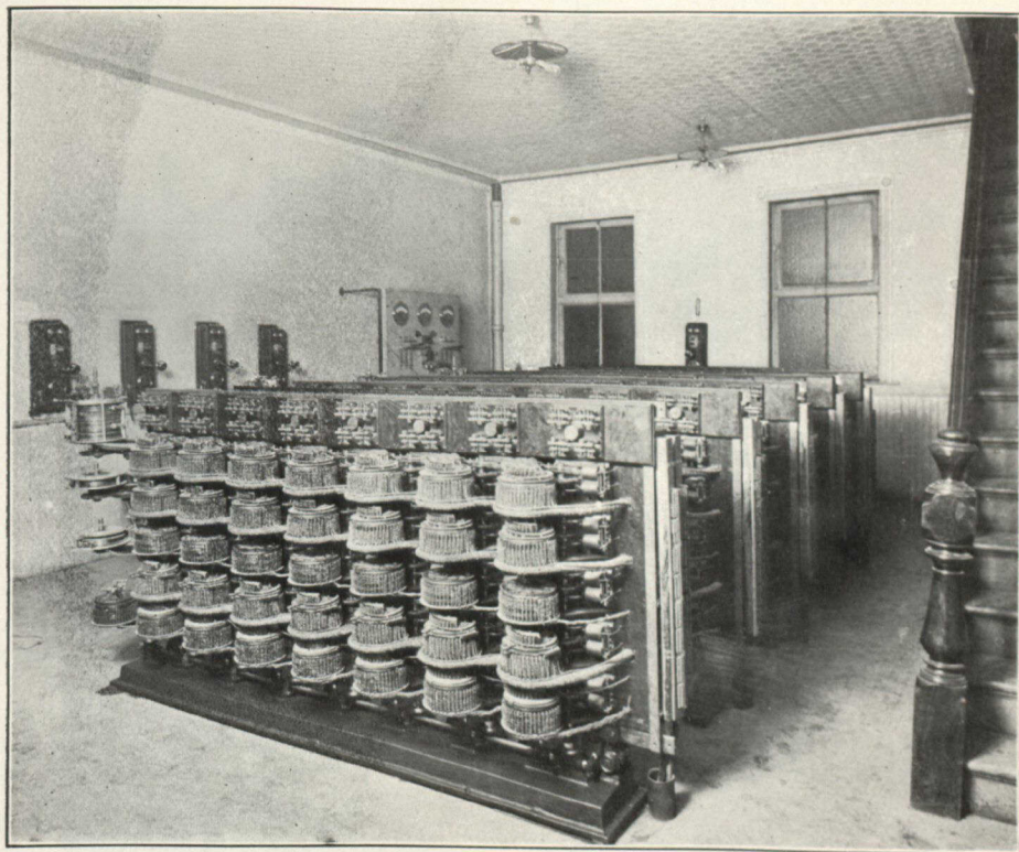
THE CANADIAN MACHINE COMPANY'S EXCHANGE ROOM AT PETERBOROUGH, SHOWING THE MACHINES THAT DO THE GIRLS' WORK AT "CENTRAL"
