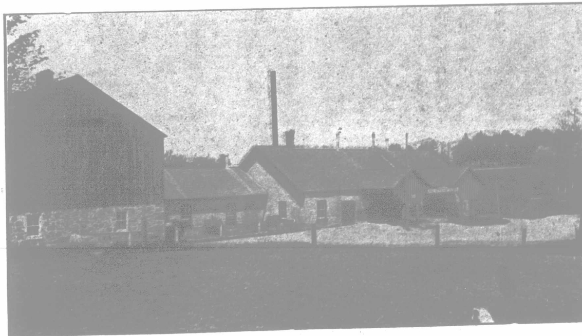
Innerkip Cheese Factory and Curing Room.
