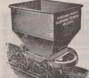
69—R. H.'s Improved Steel Hopper Wagon with Slide Door
