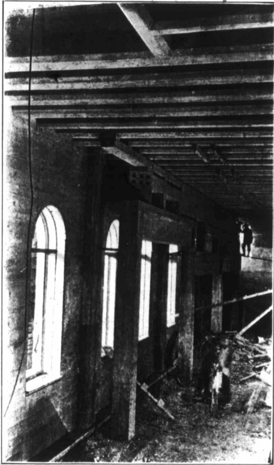
Pump Chamber and Duct System.
