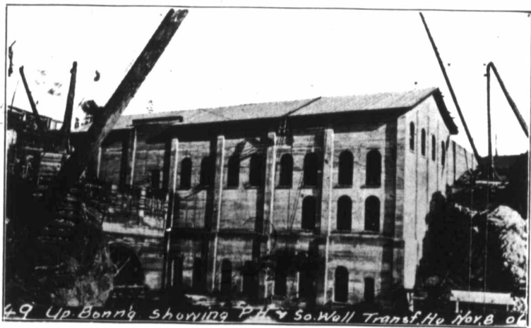
Downstream View of Power House.
