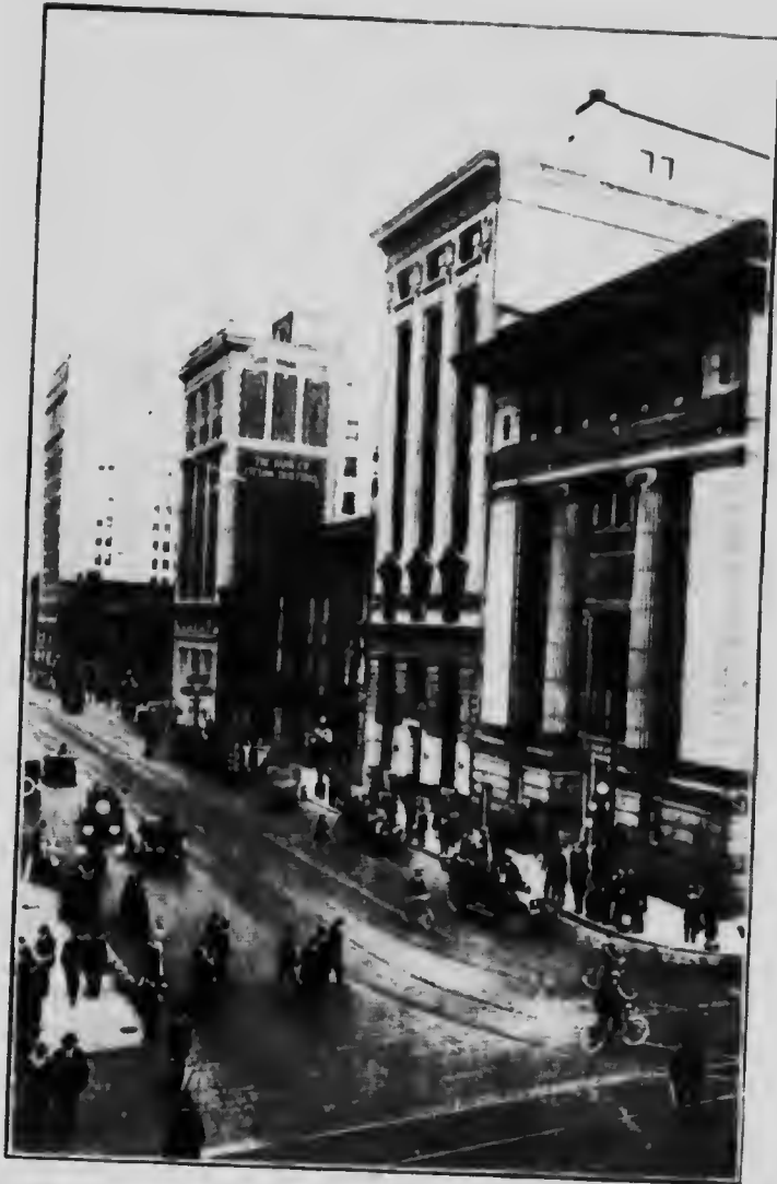
Canadian Pacific Railway. HASTINGS AND GRANVILLE STREET, VANCOUVER, BRITISH COLUMBIA.
