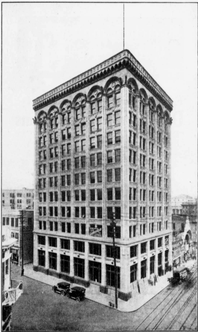
ELECTRIC RAILWAY CHAMBERS
