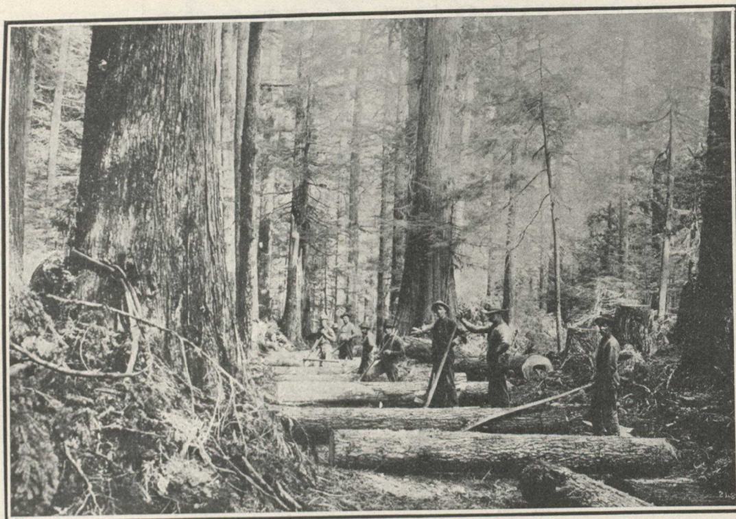
Making a skid road, over which the logs are drawn out of the bush.
