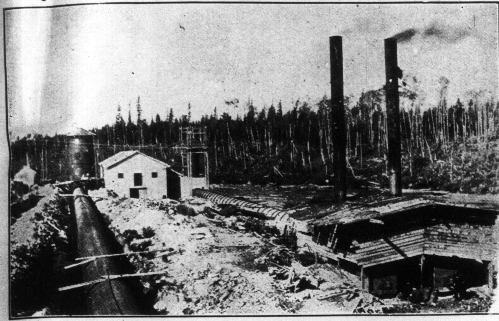
Completed Surge Tanks on Penstocks, During Construction at Sandy Falls.
