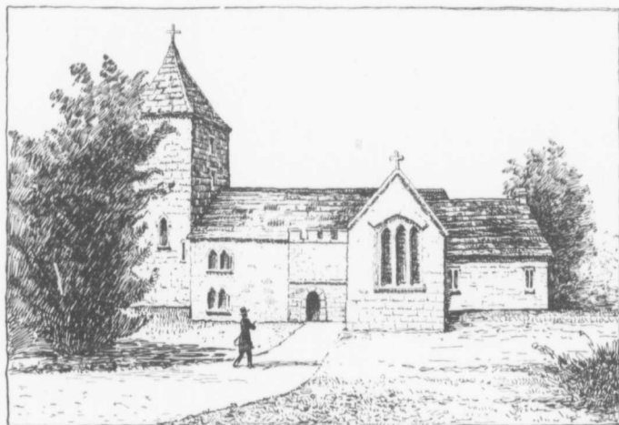
DUNKESWELL PARISH CHURCH BEFORE RESTORATION.
