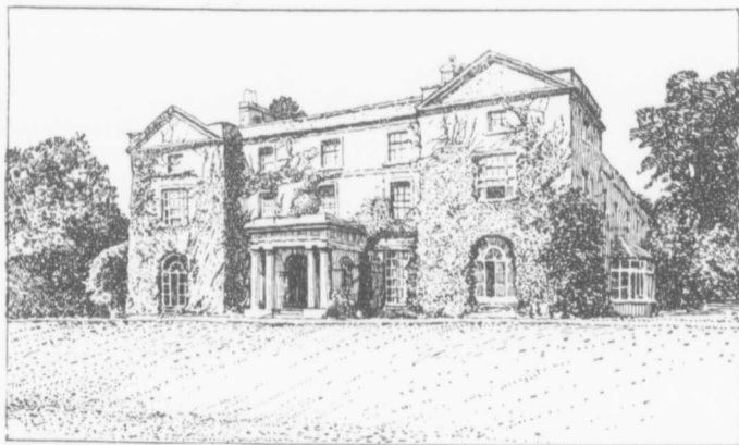
THE RESIDENCE KNOWN AS HEMBURY FORT.
