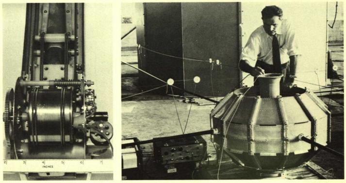
Alouette I, launched in 1962, had two antennas. Each consisted of two poles extended at right angles to one another. Each pole was stored as a tape on a spool (left) during launching. In space, as the tapes unwound, their edges curled tightly together to form semi-rigid tubes. The antennas, shown in tests (right), measured 46 and 23 metres from tip to tip. Later Alouette and ISIS satellites had 73-metre antennas.
