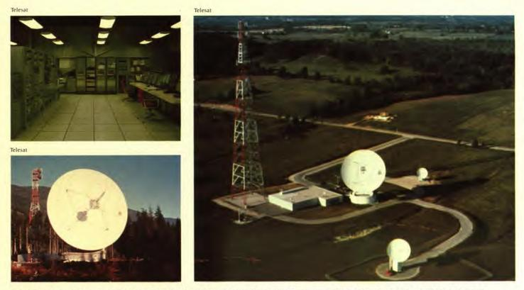
Telesat's two control stations at Allan Park, Ontario, (right and top left) and Lake Cowichan, British Columbia, (bottom left) have 30-metre antennas. The three smaller antennas at Allan Park provide tracking, telemetry and command functions. The satellite control system developed by Telesat has been used in the United States, Indonesia and Brazil.
