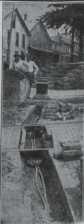
Laying STANDARD Steel-Tape-Armored Cable Across a Street.
