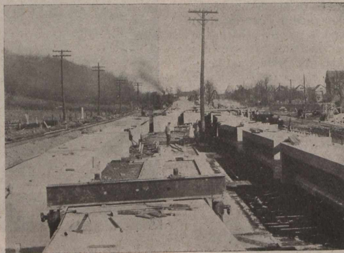
Pouring the Pre-moulded Concrete Slabs
