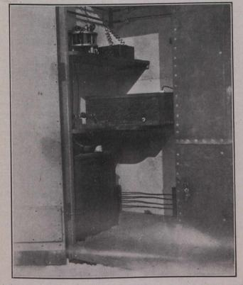
Interior Generation Box, Showing Transformer and Oscillators.
