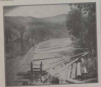
Rudder Beam, Thompson River, B.C. Notice How the Fins or Rudders Set Beam Diagonally Across Stream.
