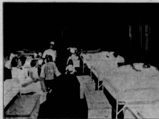
Going to bed in the International Sunshine Cottage
