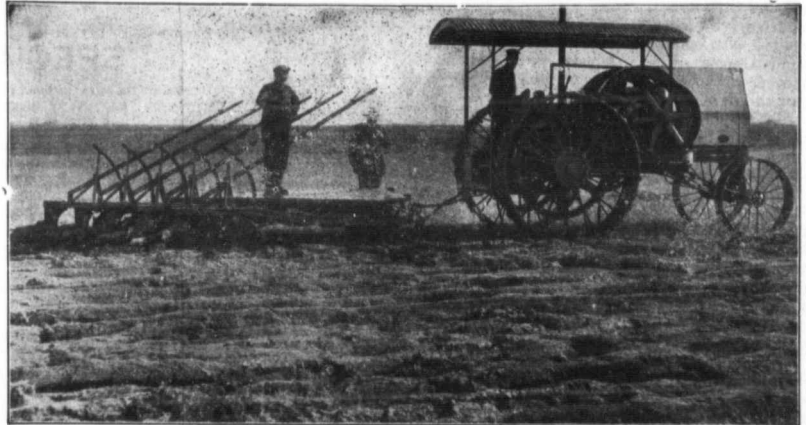
BREAKING WITH A 15-30 FAIRBANKS-MORSE TRACTOR.
