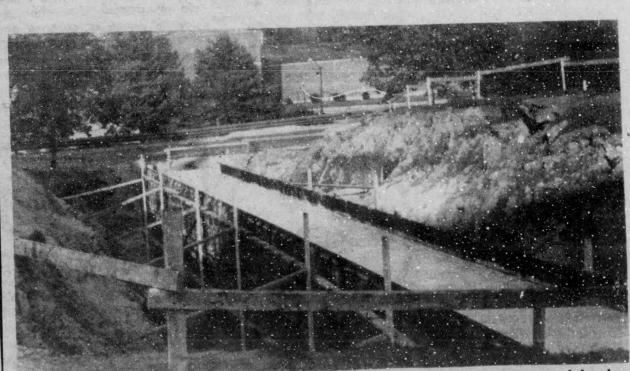
To cure the problem of leaky steam pipes leading to the Lady Beaverbrook Gym, Work has been going on over the last few weeks to install a new tunnel. The work should be finished by the end of October, but while it is in progress it will be necessary to close the road for a while in the next cou-Timothy Lethbridge PHOTO
