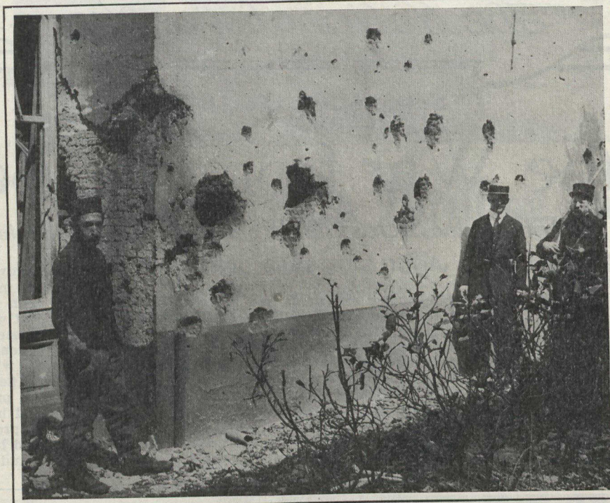
Showing how an air-flung bomb, when it burst in Antwerp, blew holes in a brick wall over a foot thick, ten yards from the point of explosion.
