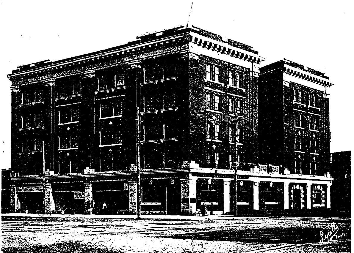
Cassa Loma Block, Winnipeg, Manitoba. J. H. G. Russell, Architect.
