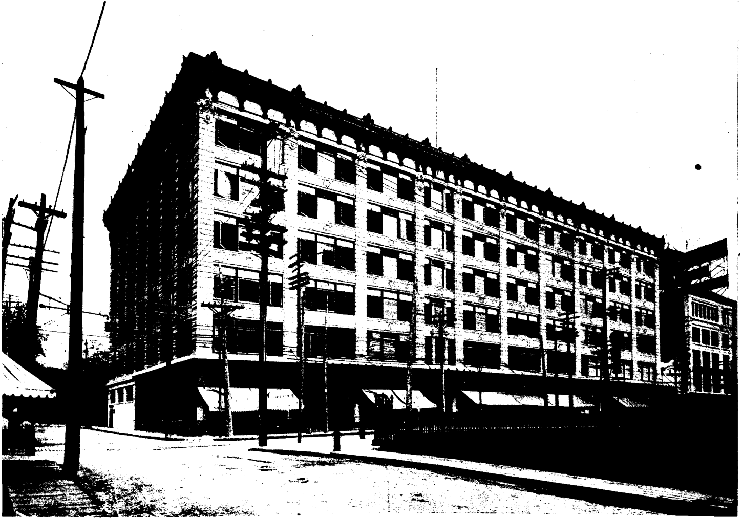
Jacobs Building, Montreal. Equipped with Standard Ideal Ware. Mitchell & Creighton, Architects. W. J. McGuire, Plumber.
