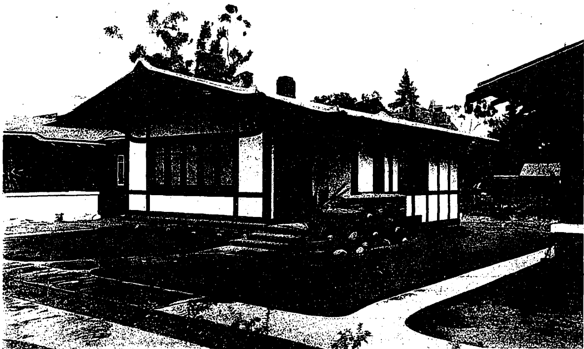
A California Bungalow at Los Angeles. Arthur Hiniman, Architect. Photo by Graham Photo Co.
