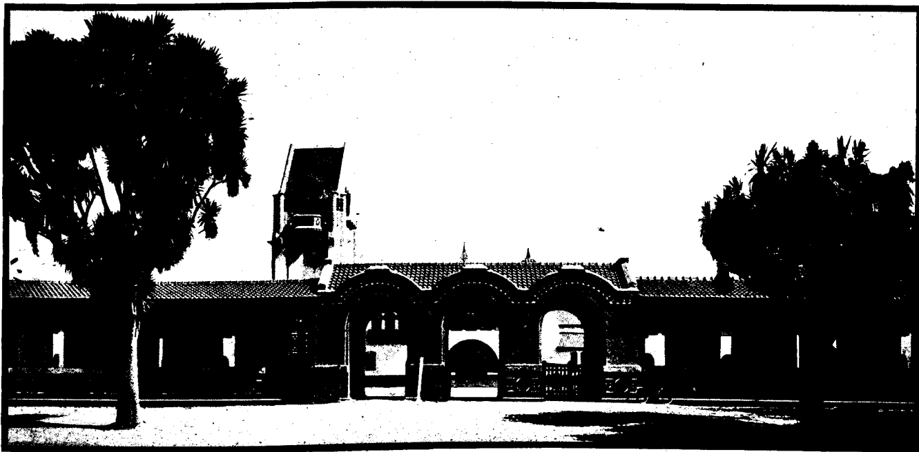
California State Normal School, San Jose, Cal., U.S.A. Largest concrete building of its kind in the world. Exterior of rough walls are covered with a pebble dash of "Medusa" White Portland Cement.
