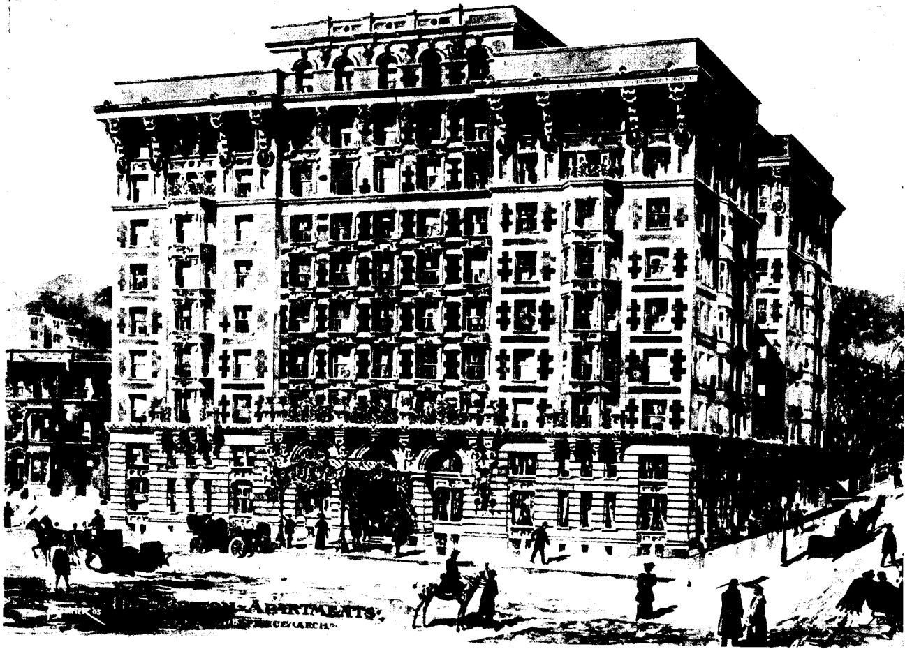
Linton Apartments, Montreal. Finley & Spence, Architects. Thomas O'Connell, Plumbing Contractor. Fitted throughout with Standard Ideal Ware.
