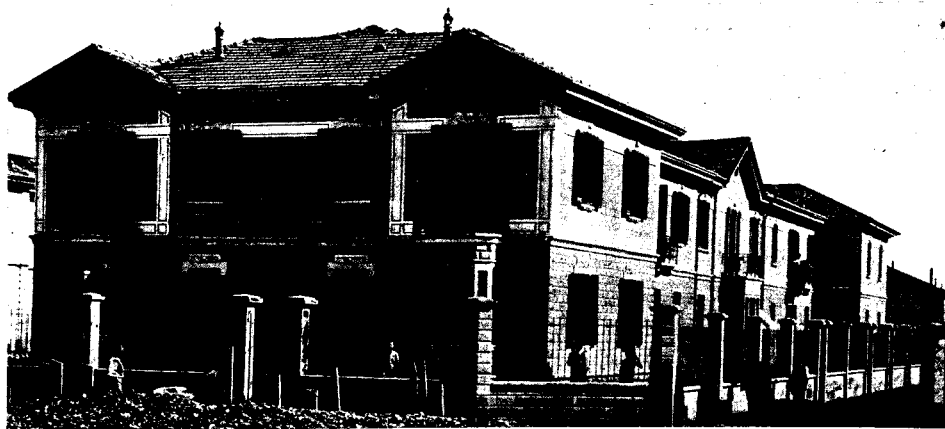
Italian Flat erected in Milano, Italy. 46,000 Concrete Blocks made on Ideal Face Down Concrete Block machines were used in its construction.
