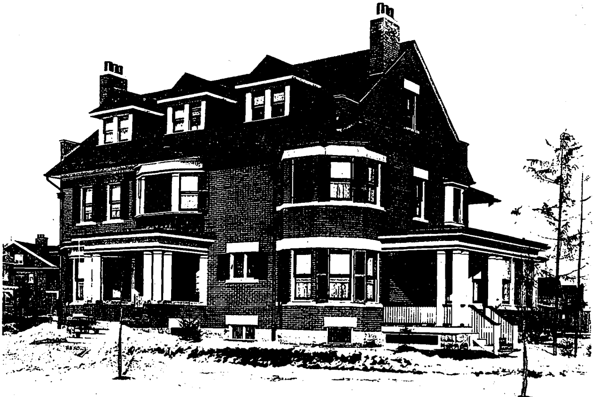
Residence of J. Donogh, Toronto, Ontario. F. S. Baker, F.R.A.I.C., Architect.
