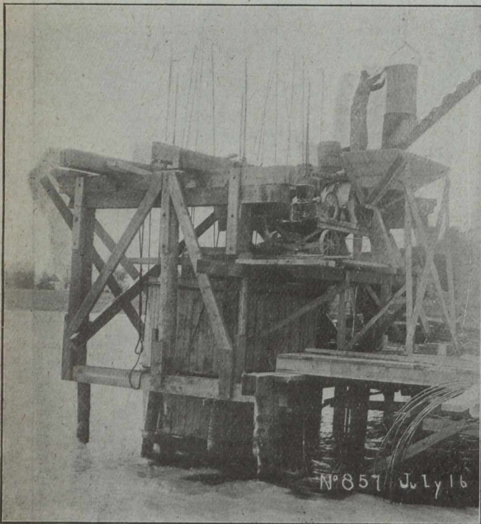
Concreting a 6 ft. Caisson Lift
