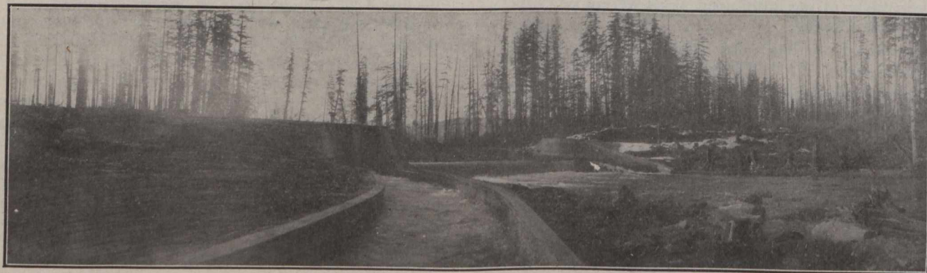
Diversion Dam with Beginning of Masonry-lined Canal. Note Fish Ladder on Right.
