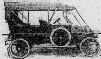
are fitted with all the latest and best improvements, including steel detachable wheels, worm or bevel driver, four forward speeds and reverse, foot accelerator, etc.
