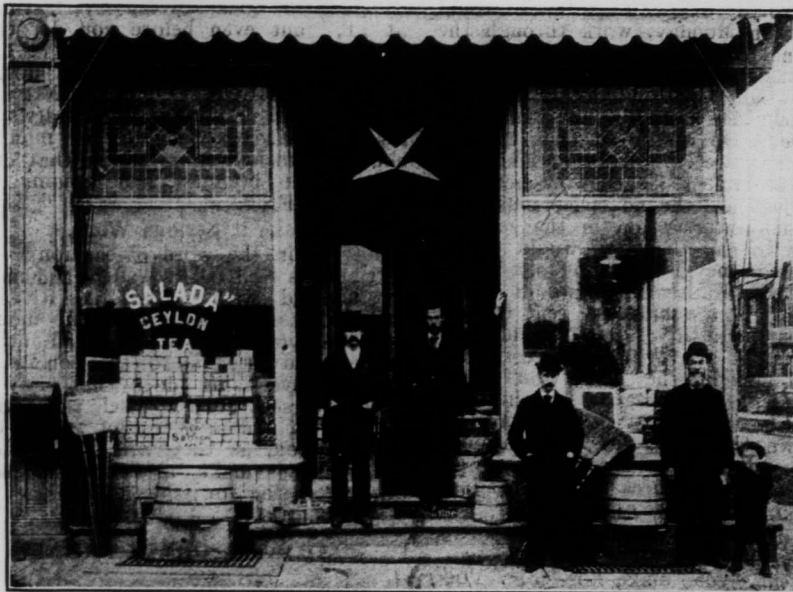
One of the first window displays ever made for "Salada" Tea. Taken in 1893—over seventeen years ago.
