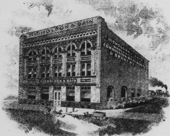
BANNATYNE ST. EAST TRANSFER TRACK.
