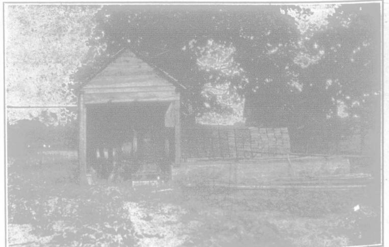
Cement Storage Tank and Pumping Outfit for an Overhead Irrigation System.
