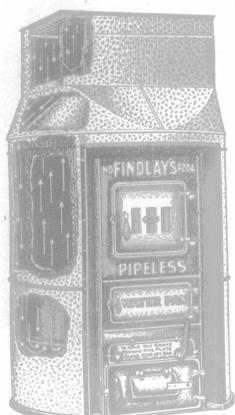
Will not heat your cellar. No pipes to take up important space. No tearing up of walls and floors for registers.
