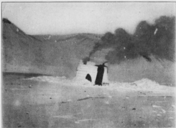
The blacksmith's shop, March, 1911.
