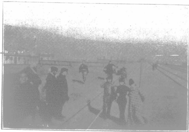
Station in Manchuria.
