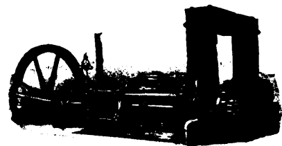
Cross-Compound Corliss Compressor
