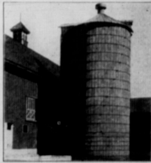
Concrete stave silo. There are a few of these in Manitoba and they have given good satisfaction. Hollow stock or hollow wall concrete silos are usually but fairly best resistant and satisfactory.
