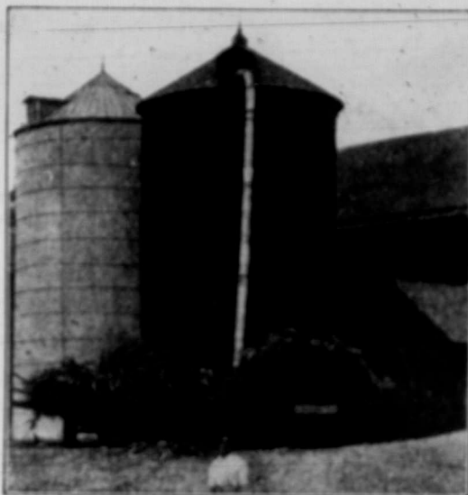
Filling a stave silo. The filling problem in a busy season is one of the most difficult, but will gradually become less so as silage growing facilities. These are wood stave silos, not too expensive and very efficient. Note the straight pipe and that the wagons are close up.
