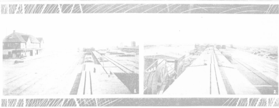
1. East View GRAND TRUNK PACIFIC YARDS 2. West View
