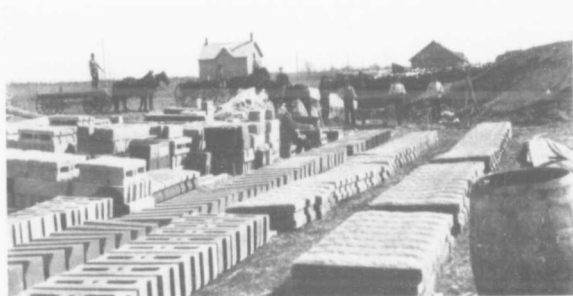
Cement blocks are manufactured in great quantities
