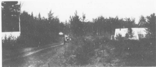
Tents of the advance guard for the Hudson Bay Railway
