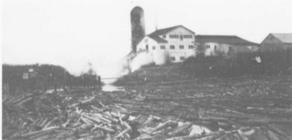
Innumerable logs demanded by a great building record
