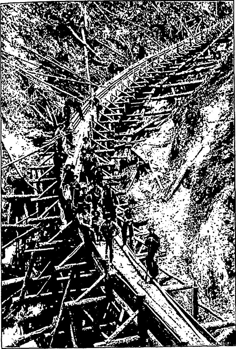
Columbia River Lumber Company, Golden, B.C.—Hanna's Camp. Slide for driving logs almost completed, 700 feet long and drop of 125 feet. Photo taken on May 10th. That night the reserve dam in the mountains burst and swept entire work away.
