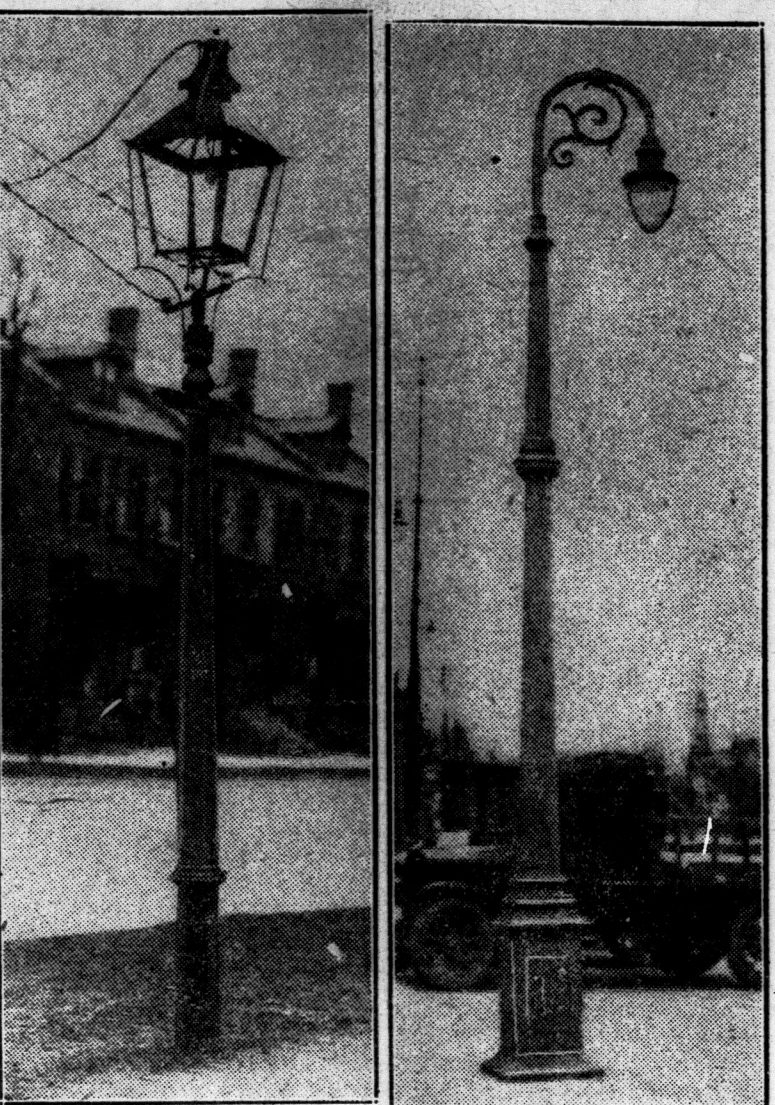
THE OLD AND THE NEW. In the past forty years, wonderful progress has been made in developing street illumination. Just how great the stride has been is strikingly indicated by the two lamp posts shown in the picture, one ancient and the other modern, and they stand on Dundas street within a short two blocks of each other. One is a post and lantern frame, a survivor of the period of gas illumination, which stands before the Congregational Church at Colborne street, and the other is an ultra-modern electric light standing before the public utilities commission building. In its palmist days the gas light boasted a power of sixteen candles; the electric light is 750 candle power.
