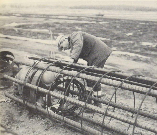
Dr. Michael Bozozuk checks the instrumentation of a steel reinforced pile, one meter (3.3 ft) in diameter and 90 meters (300 ft) long, driven during the construction of a highway overpass near Berthierville, Quebec.
