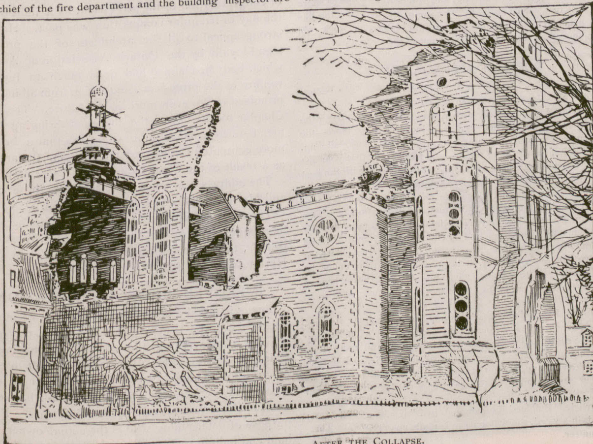
THE NICOLET CATHEDRAL, AFTER THE COLLAPSE.
