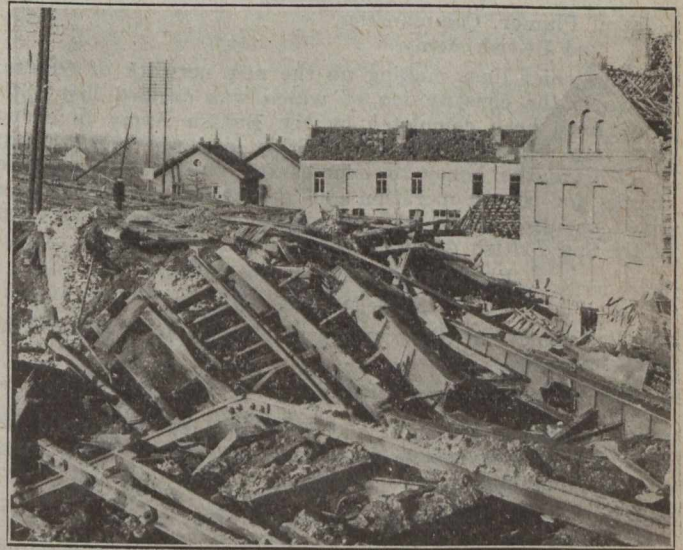
BRIDGE BETWEEN LILLE AND BRUSSELS DESTROYED DURING HUN RETREAT—REBUILT BY CANADIAN RAILWAY TROOPS
