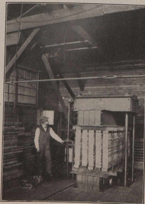
Automatic Hydraulically Operated Door-Veneering Machine.
