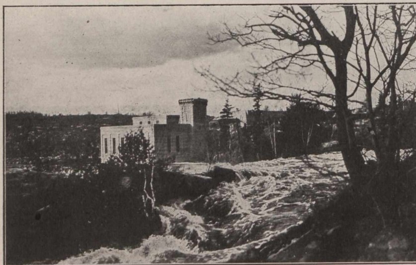
View of Generating Station.
