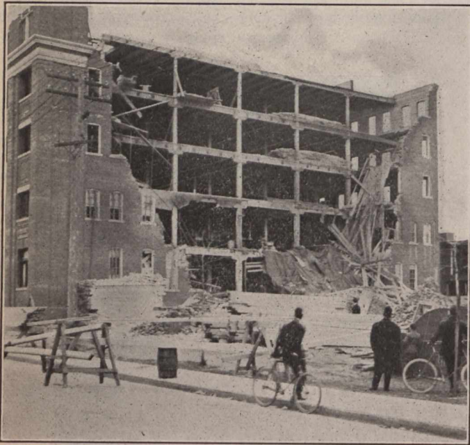
View of Building After Collapse of Wall.
