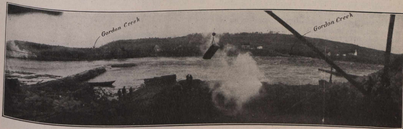
Fig. 1.—Timiskaming Dam, November, 1910. Coffers Dams, Quebec Channel, Stopped by Autumn Floods.
