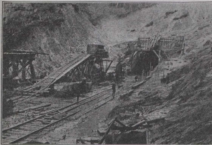
Portal of Tunnel 3 During and After Construction, Showing Troublesome Material Encountered.
