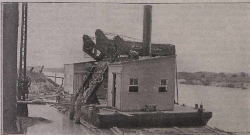
Fig. 2. Gate Lifter, with top of derrick lowered for passing under bridges.
