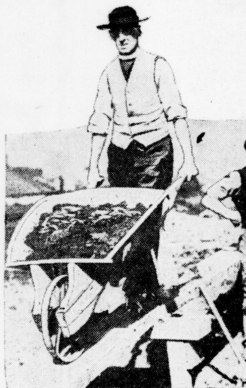
Rev. D. J. Morgan, vicar of a church in South Wales, is acting as a laborer in the excavation work preparatory to the building of a new church. He was aided by sixty of his congregation
