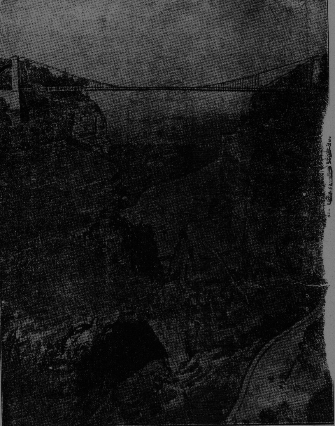
A marvellous feat of engineering skill performed by French engineers at Constantine, French Africa. The bridge is suspended at a height of more than 300 feet over the Rhummel river and runs between sheer precipices of chalk cliffs on each side. Owing to the difficulty of approaching the work this is regarded as the greatest piece of engineering work yet completed. It is regarded as a much greater achievement than the Niagara suspension bridge, because of the fact that the supports had to be imbedded in the solid rock, and because of its great height above the valley level. This bridge is the first of its kind in the world. It is the longest bridge of its kind in the world. It is the longest bridge of its kind in the world.
