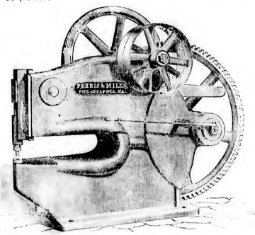
POWER PUNCHING MACHINE, EXHIBITED BY FERRIS & MILES IN MACHINERY
