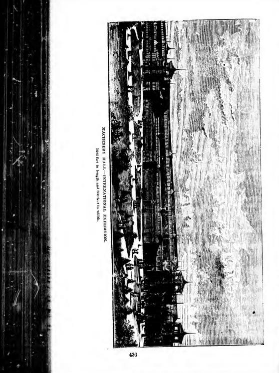
sash are movable for ventilation. Louvre ventilators are introduced in continuous lengths over both the avenues and the aisles. The building is lit entirely by side light, and stands lengthwise nearly east and west."
