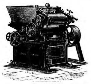
FOUR-CYLINDER SOAP-MAKING MACHING EXHIBITED IN THE FRENCH SECTION, MACHINERY HALL.
