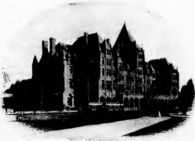
CANADIAN PACIFIC RAILWAY COMPANY'S PLACE VIGER HOTEL AND STATION, MONTREAL.
