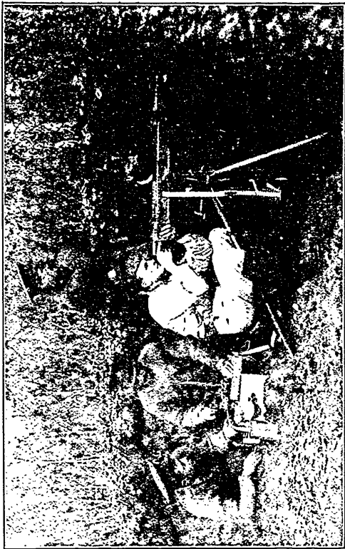
Frontispiece:—A hasty emplacement excavated in a fold of the ground. Note leaves spread about to conceal fresh-turned earth from observation.
