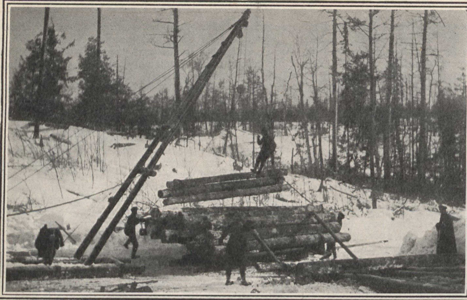
Loading a Sleigh from a Skidway by a Steam Crane.
