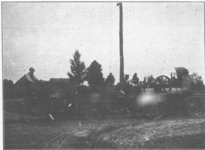
OPERATING THE GRADER BY MEANS OF THE TRACTION ENGINE
