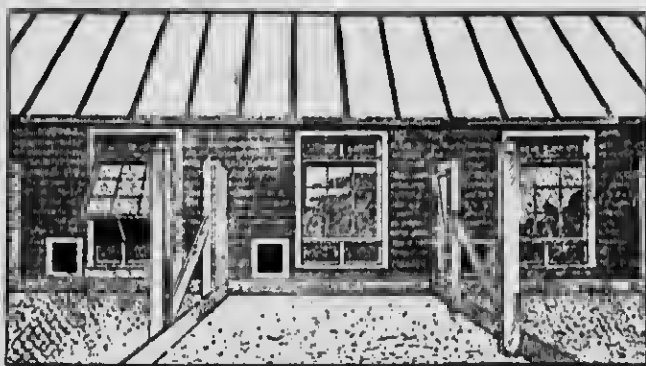
Outside—This Illustration Shows the Door and the Cotton Panels, Above and Below the Window in the Peerless Poultry House.
