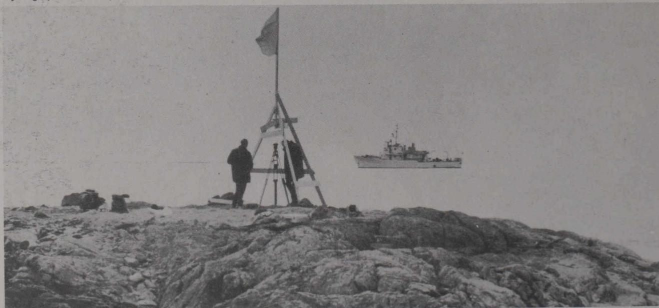
Hydrographic control point on the shores of Newfoundland: CSS Maxwell in background.
