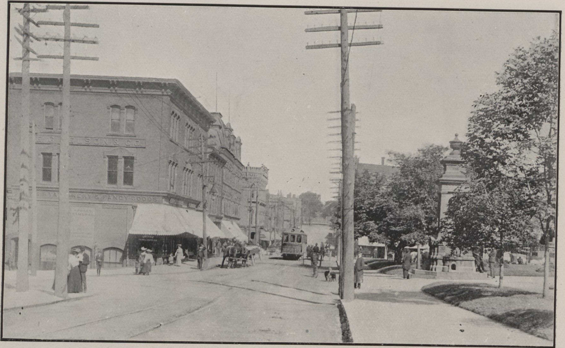
VIEW OF CHARLOTTE STREET—ST. JOHN, N.B.
