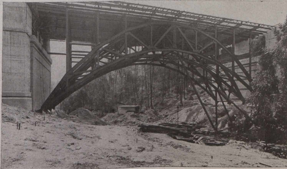
Fig. 7.—Rosedale Section, Bloor Street Viaduct, Looking South Along Ravine Drive.
